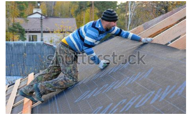
7. moisture barriers in construction,
