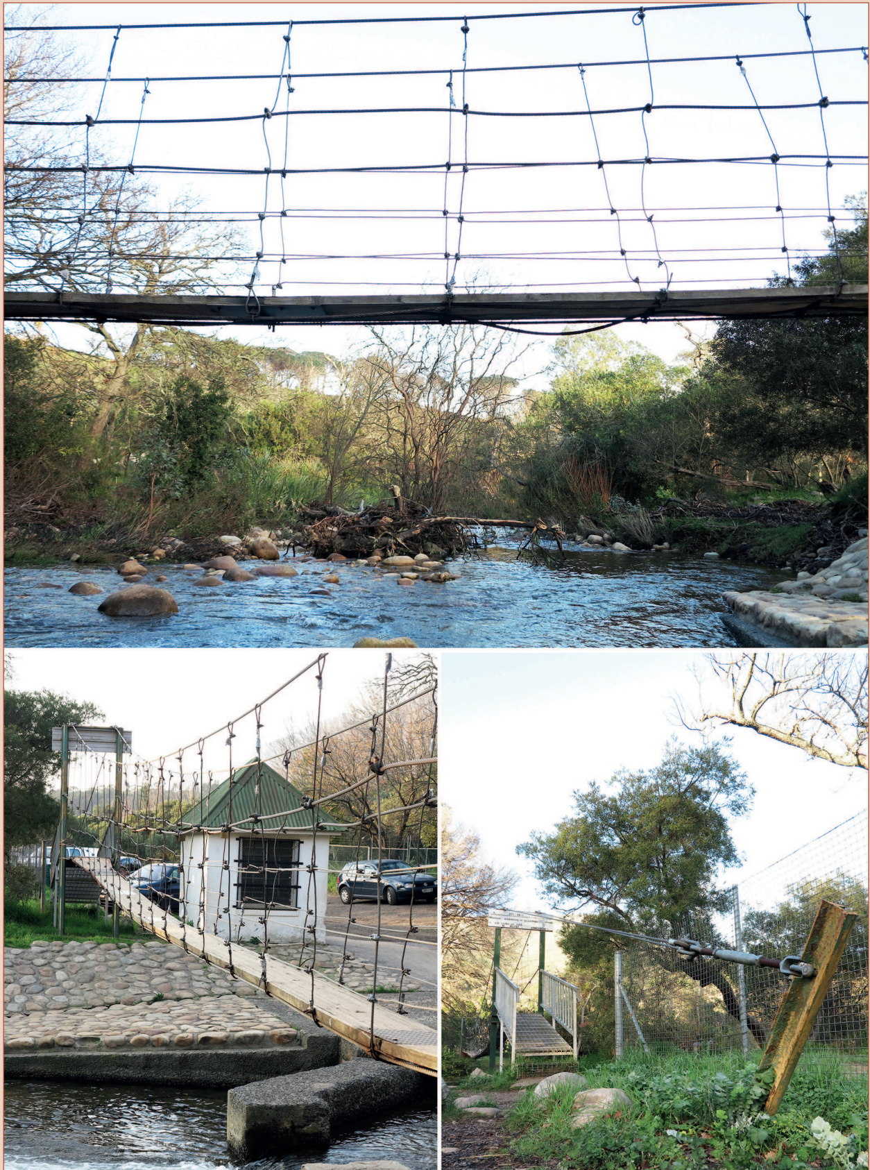
Figure 3: What is this structure for? How is it supported?
