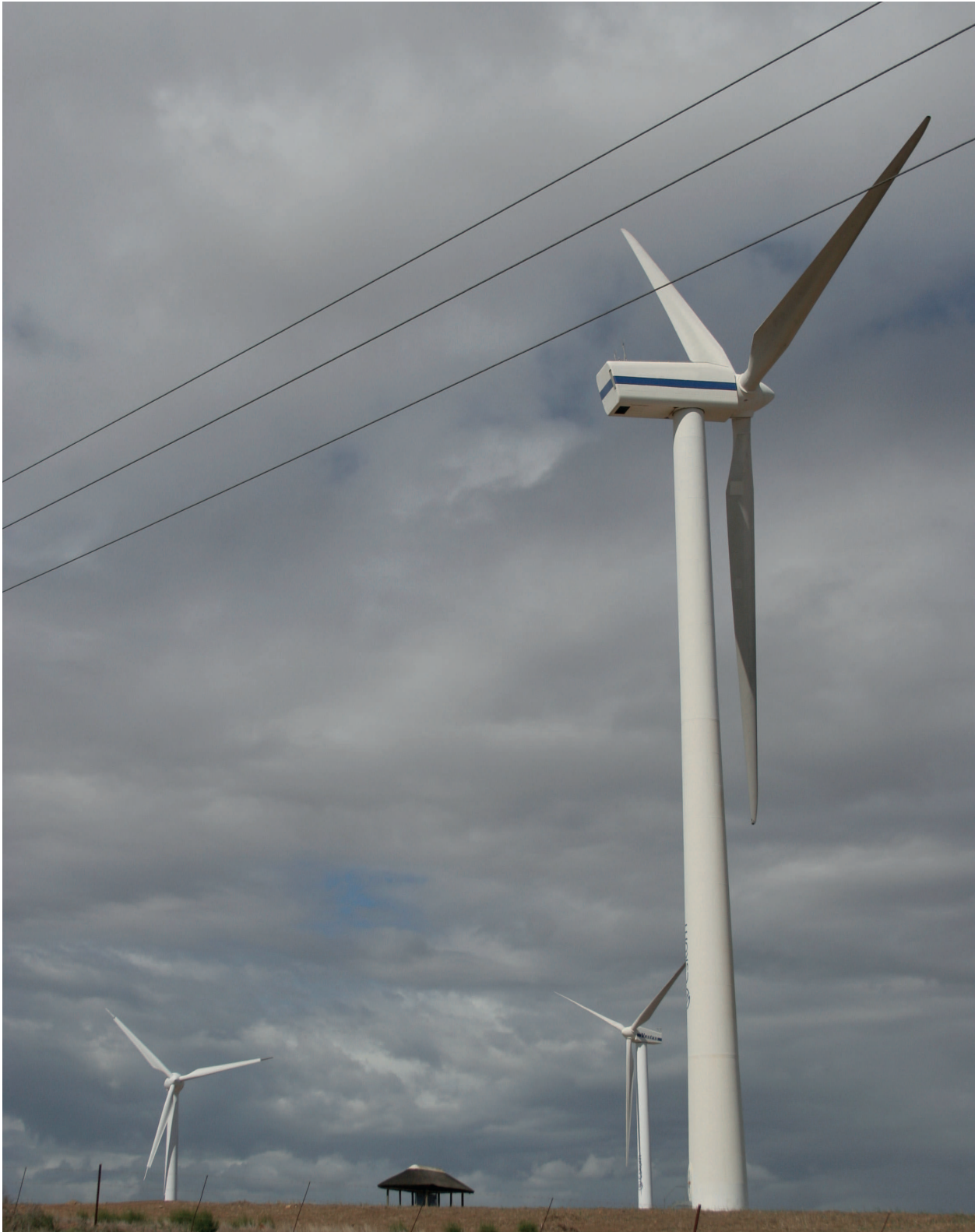
Figure 8: A wind turbine generates electricity by using the force of the blowing wind. The blades of the turbine are made of a synthetic material called “epoxy resin,” that is combined with fibres. This makes the blades very strong, but at the same time very light. Also, it is possible to make this material into a special shape.
