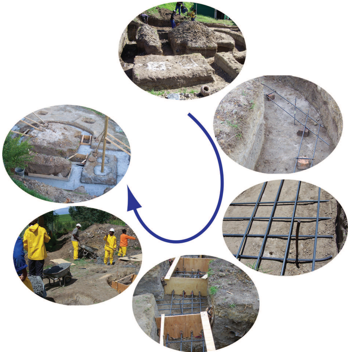
Figure 18: Steel reinforcement is used to strengthen the concrete foundations of a new house.
