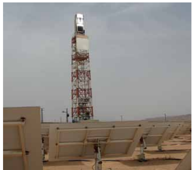
Figure 10: Mirrors in a solar-powered power station focus light onto heating towers.
