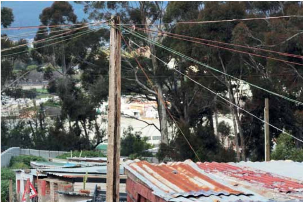
Figure 7: Illegal electricity connections in an informal settlement. Notice that there is no control box at the top of the pole for measuring electricity usage or for cutting off the electricity in case of a short circuit.
