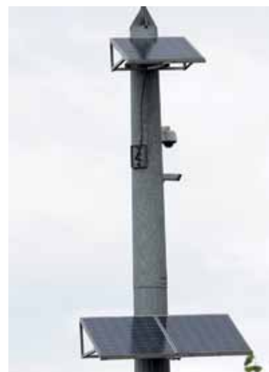
Figure 14: Photovoltaic cells on a pole
