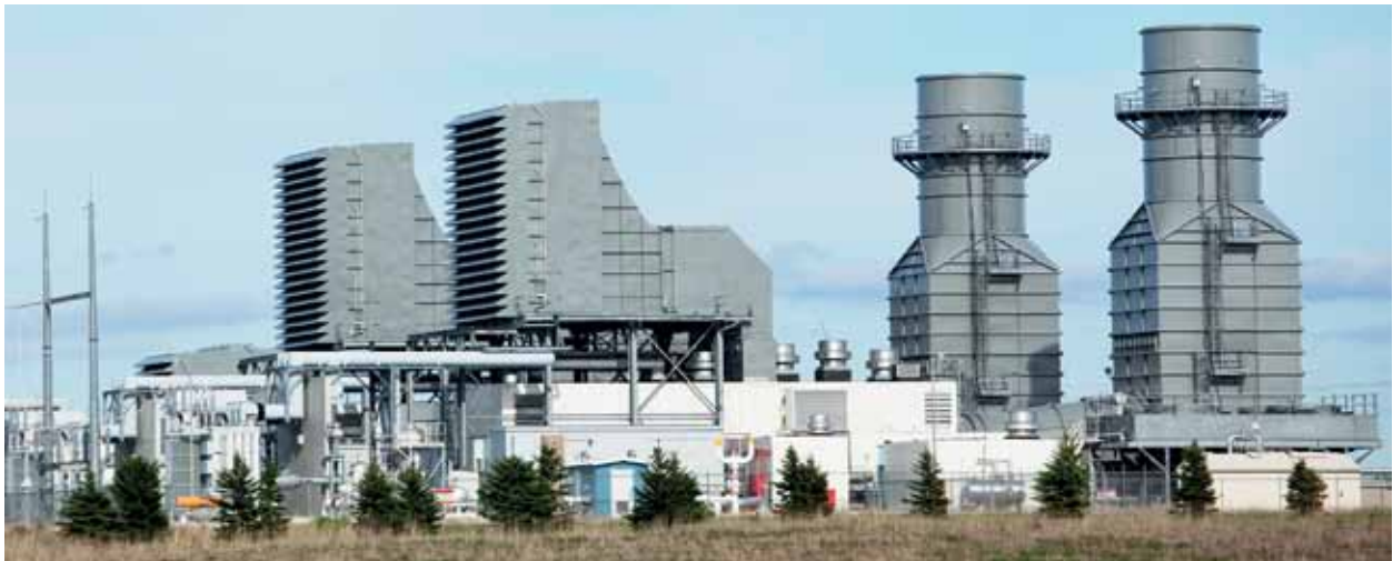
Figure 7: A gas-turbine power station
