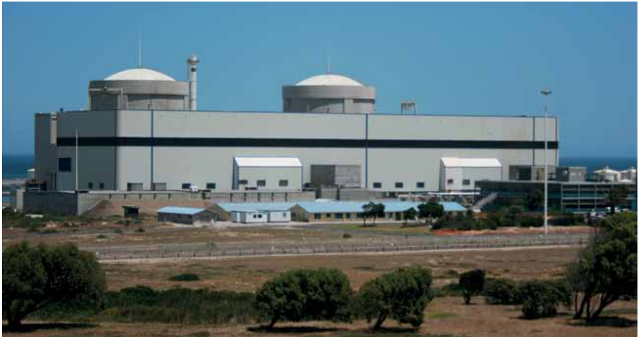
Figure 8: A nuclear power station
