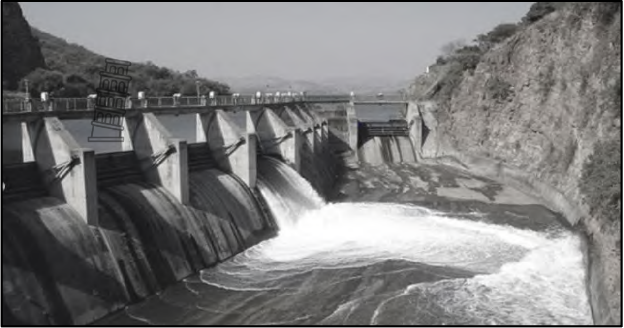
FIGURE 3.6: HARTBEESPOORT DAM WALL
